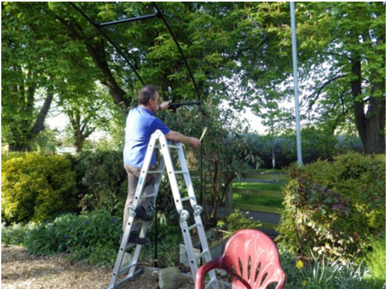
John erecting the new entrance arch into the Sensory Ride
